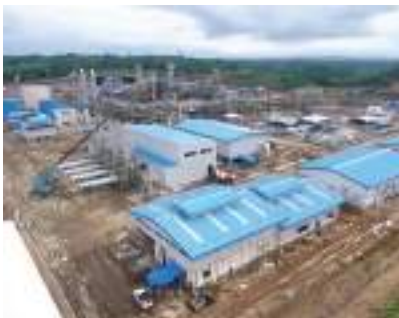
ME WORKSHOP, MAIN CONTROL ROOM & HAZARDOUS WASTE BUILDING
